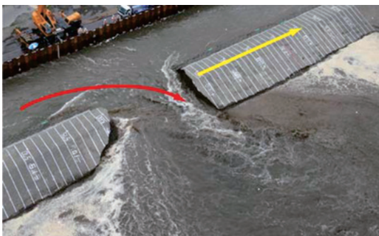
図-8 Step3 [拡幅加速段階]
