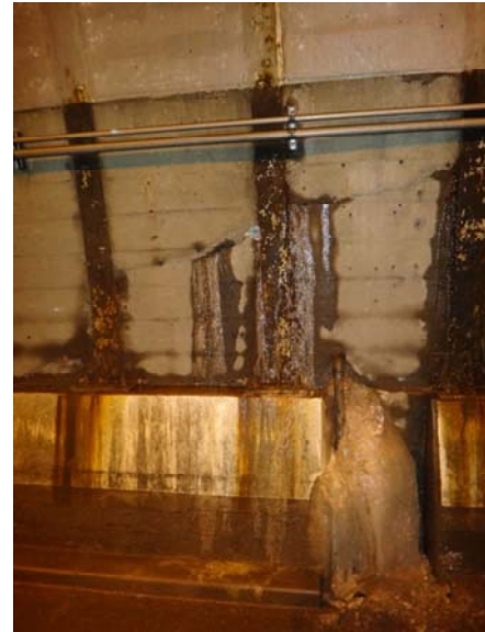
図-11 坑壁の溶食
