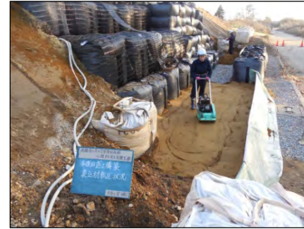
④裏込材敷均し・転圧
