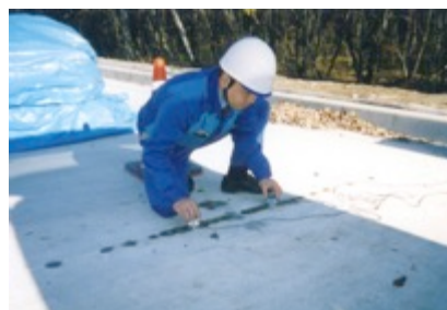
Figure 5: Measurement of the velocity of ultra-sonic wave in concrete
