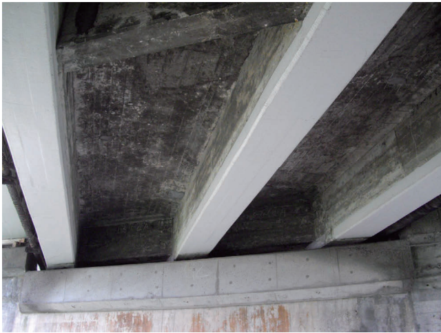
(a) 橋梁外観
