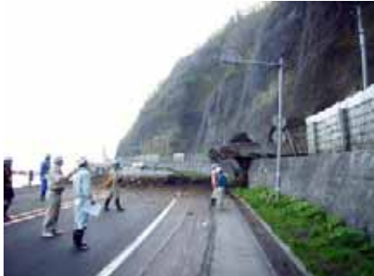
PWRI's researchers conducting investigation at the seaside rock collapse disaster site of Oshoro, Otaru-shi. area by returning the benefit of research
