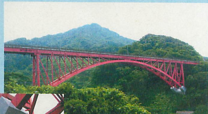
A long span bridge that did not suffer damage during the 2007 Niigata-ken Chuestu-oki earthquake (Mj6.8) because of seismic retrofit guided by the PWRI.
