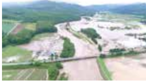
Levee breach by overflow beyond the designed level
