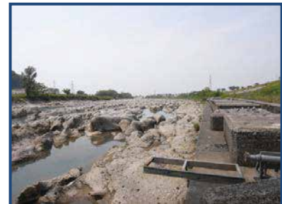
Lowering the riverbed/exposed bedrock
