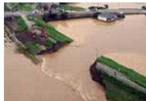
Levee breach by piping
