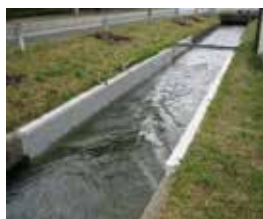
Example of waterway repair
