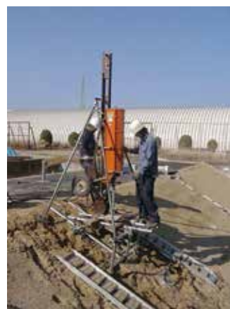
Photo of the device being installed
