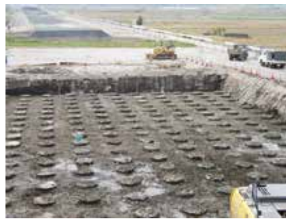
Soil improvement work at Maibara Bypass
