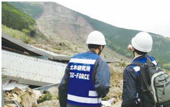
Kumamoto Earthquake: Field survey of the collapsed Aso-Ohashi Bridge and the landslide on the national highway No.57 (17 Apr.)
