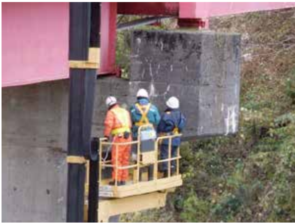
A road maintenance technical team assessing the earthquake resistance of a bridge
