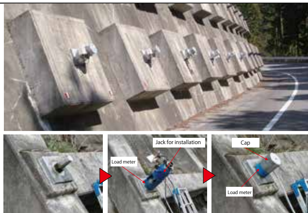
Installation of the technology
