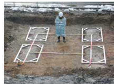
Soft ground countermeasure work at the Maruyama River
