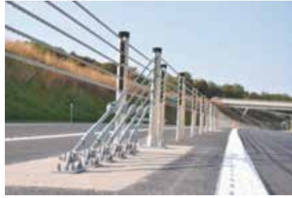
The wire rope-type protective fence
