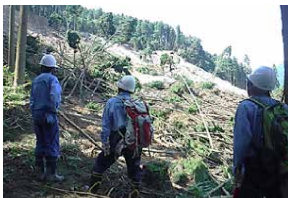
Northern Kyushu heavy rain: investigating landslide damage at a collapsed roadside slope (photo taken on July 13, 2017)
