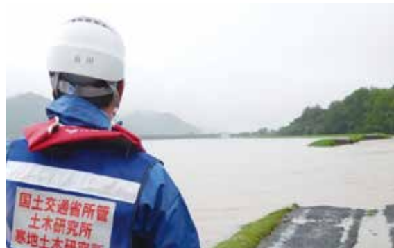
Typhoon No.10 etc.: Investigation of the overflow and the collapse of embankment in Kitami City (21 Aug.)
