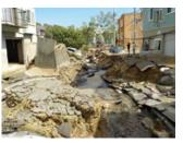
Liquefaction damage in a residential area
