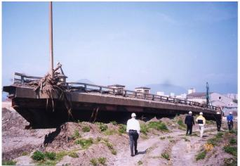
Figure 7. Bridge Washed Away by Mudflow.
