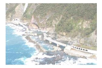
Figure 2. Washout of Four Spans of Oomori Bridge
