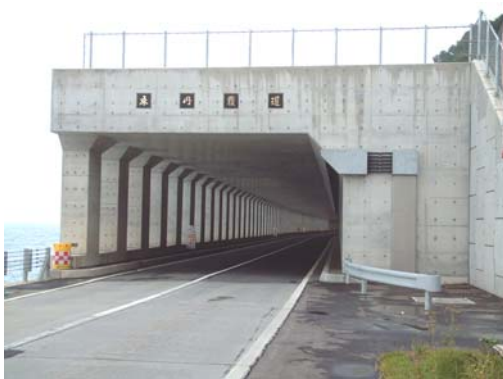
Photograph 1. Reinforced Concrete Rock Shed
