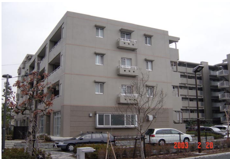
Figure 6a. Base-isolated structure in Japan
