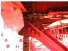
Photo 2. A large-span steel girder and truss bridge used in the autopsy survey and corrosion of its typical gusset plate.
