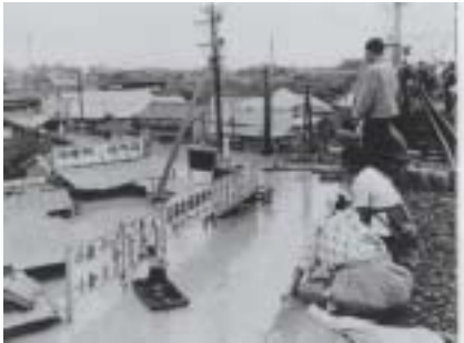
Photo-1: Flood in Tokyo due to Typhoon Kathleen
