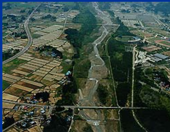
Riverside forest to decelerate flood and prevent mud flow intrusion
