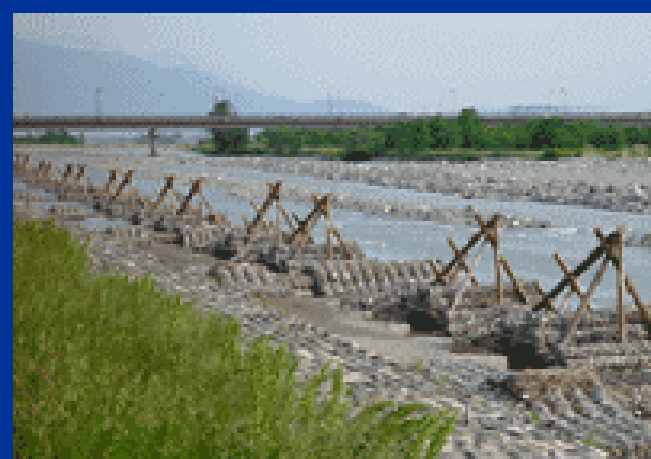
Traditional groin to encounter against flood and strengthen bank with soil and sediment
