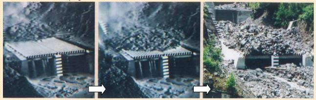
Debris-flow dewatering dam at work (Matsumoto sabo office, MLIT)
