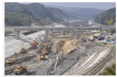
Construction of Hii river divergent channel
