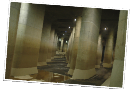
Discharge channel in Metropolitan Area Outer Underground
