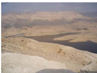
The Mujib Dam, one of the project's model sites, is located in the central part of Jordan
