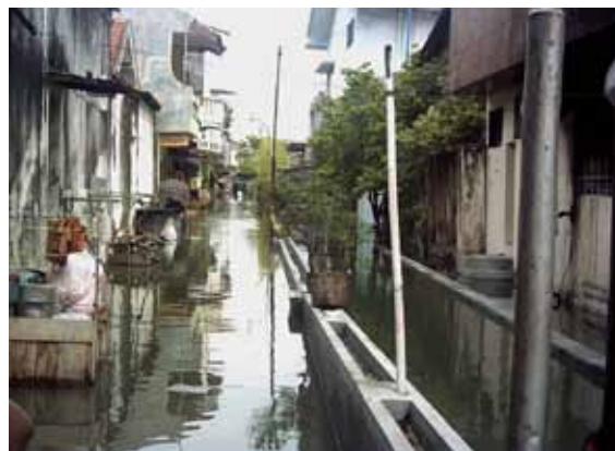
Flooded area in Solo (2007 flood, taken by BBWS Solo.)
