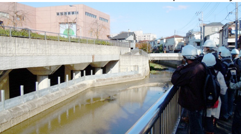
Shirakogawa River Underground Regulating Reservoirs
