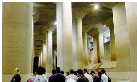
Metropolitan Area Outer Underground Discharge Channel
