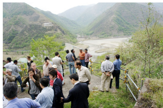
Ashio Sabo Dam
