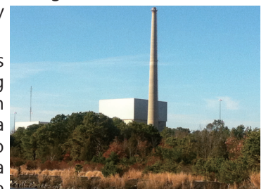
Photo2: Oyster Creek nuclear power plant in New Jersey
