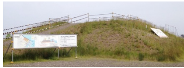
Sample levee to show local residents how high the new levee will be.
