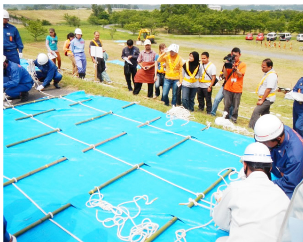
A demonstration of a flood fighting method using a water-proof sheet
