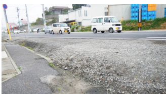
Heightened road near the Kesenuma Fish Market
