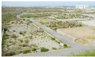
View from the higher ground towards the Natori River (Machines for seawall construction are visible in the upper right corner of the photo.)
