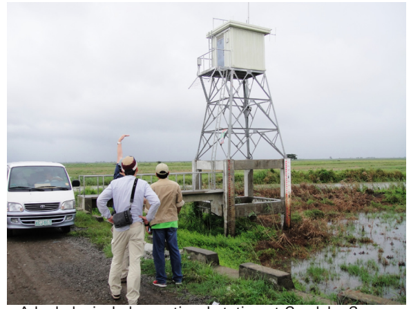
A hydrological observational station at Candaba Swamp
