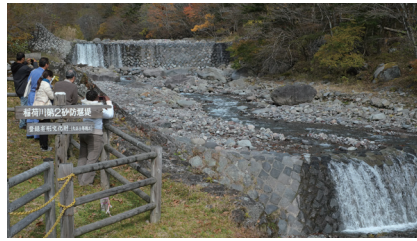
At the Inarigawa erosion control dam
