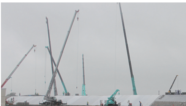
Dike restoration work in progress
