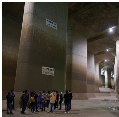
At the metropolitan area outer underground discharge channel in Kasukabe city
