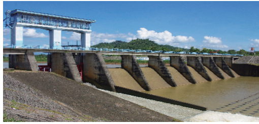
Colo Weir, a water intake weir taking irrigation water from the Solo River
