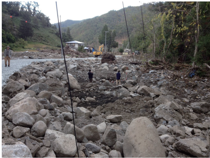
Photo 2 Damaged Horono district due to inundation.
