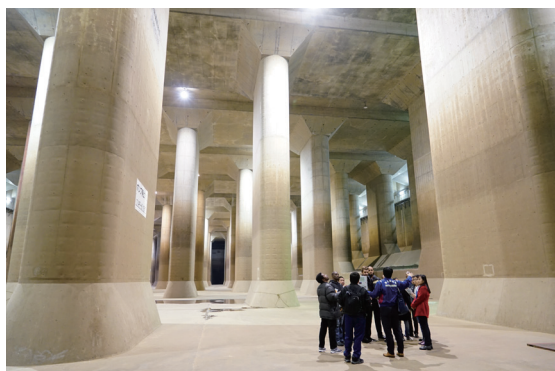
The Metropolitan Area Outer Underground Discharge Channel (Kasukabe city)
