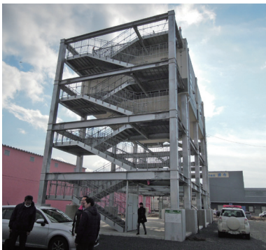
Tsunami evacuation tower
