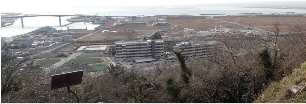
Planned site for the tsunami memorial park (the buildings on the near side were built for disaster victims)
