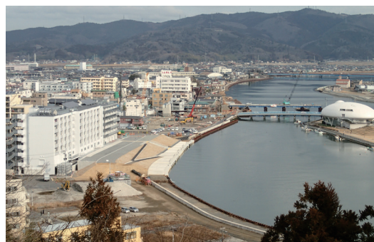
A completed section of the river levee along the Old Kitakami River
