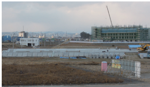
Public housing under construction
