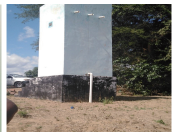
Data logger inside the DCP House- Monitoring of water levels
