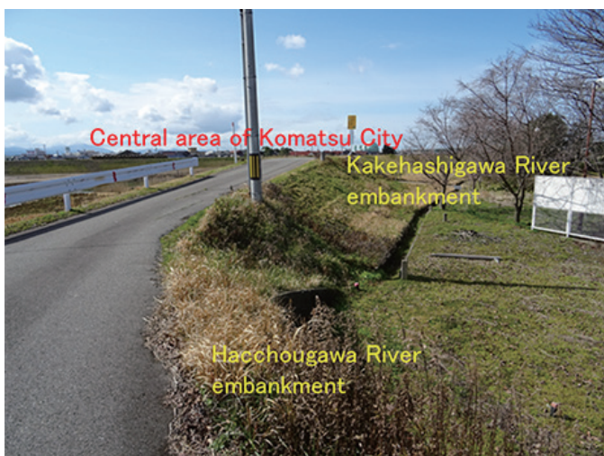
Figure 2 The downstream area of the Hacchougawa River, where the floodwaters of the Tedorigawa River may overflow and flow into the Kakehashigawa River. The central area of Komatsu City is located along the left bank of the Kakehashigawa River.
