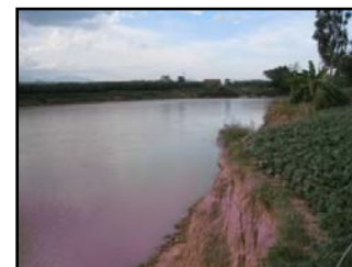
Bank erosion (Quang Nam)
