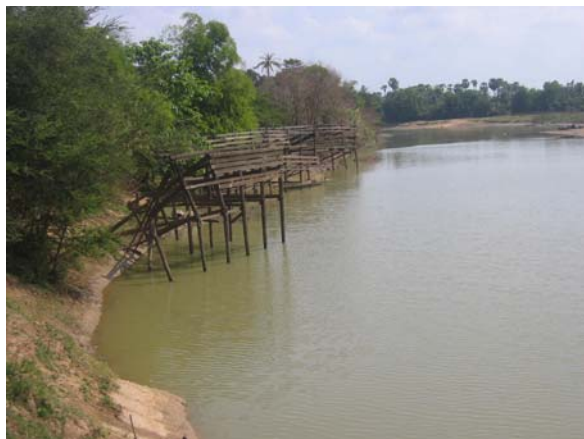
Picture 9 Wooden structures to protect bank from erosion
