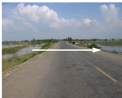
Picture 2. Spill way provided on the national road
