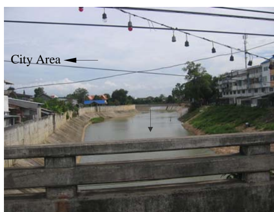
Photo 5 Levee in Uta-Pao River in Hat Yai city
