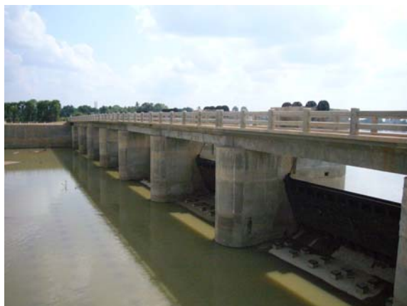
Picture 12 Barrage constructed for irrigation use
