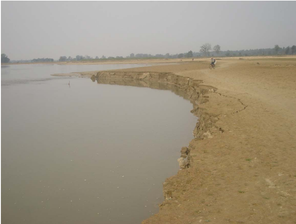
Photo 11 Bank Failure and Deposition Silt
