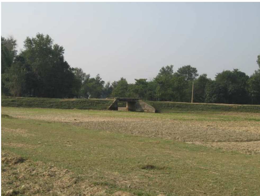
Photo 2 Cross Drainage Structure
