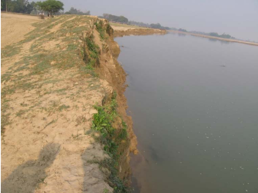
Photo 1 General View of River and Bank Condition
