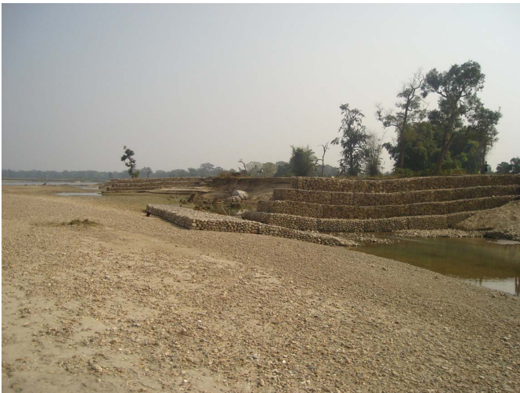
Photo 8 Series of Spurs for Protection of River Bank and Cultivated Land
