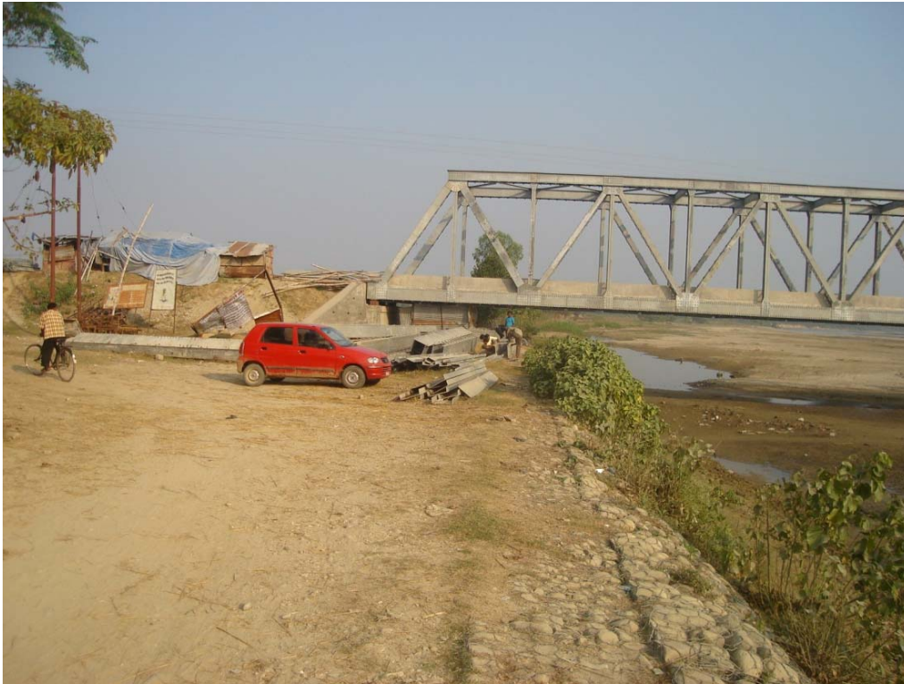
Photo 5 Steel Truss Bridge with Bank Protection Still Under Construction Since 1997
