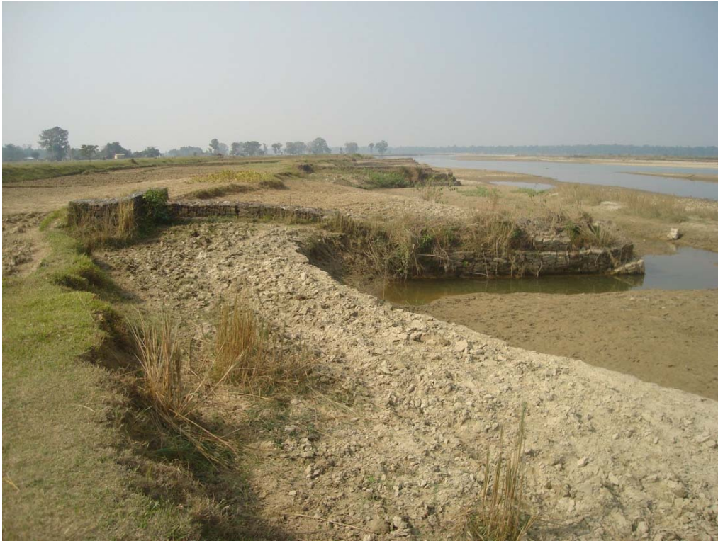
Photo 7 Protection of Cultivated Land with Spur
