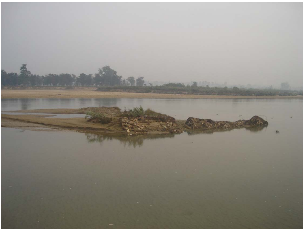
Photo 10 Failure of Spur
