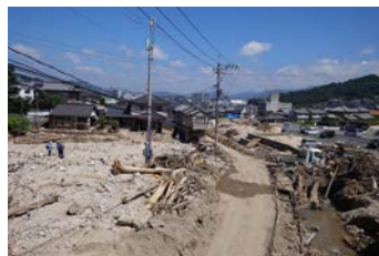
An area along the Souzu River in Saka Town, Hiroshima Pref., Japan, severely affected by a flood with a massive amount of sediment in July 2018
