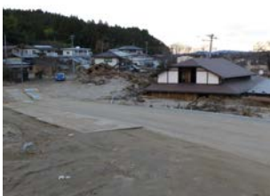
A house half-buried in a massive amount of sediment after a flood event that hit Marumori Town, Miyagi Pref., Japan, during the passing of Typhoon Hagibis in September 2019.
