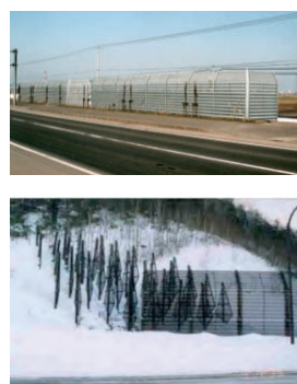
図-5 防雪柵の端部対策例
