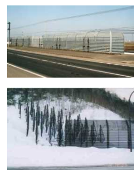
図-5 防雪柵の端部対策例
