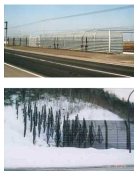
図-5 防雪柵の端部対策例
