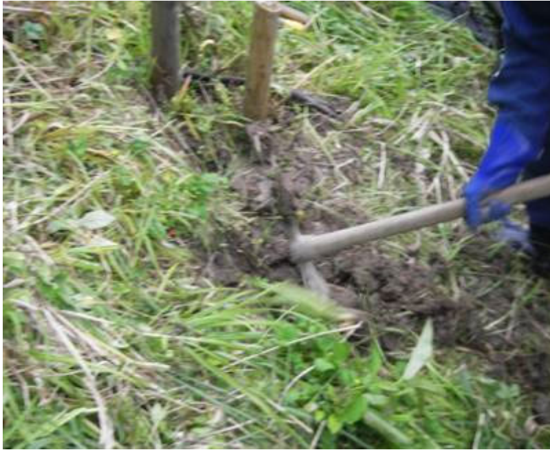
設置斜面掘削
