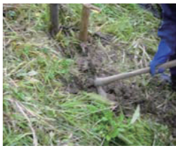
設置斜面掘削
