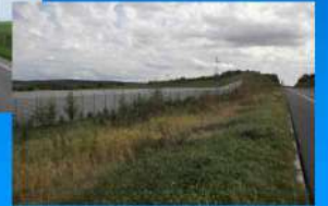
緩勾配盛土 (R40豊富BP)
