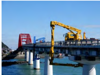
橋梁点検・診断
