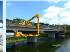
橋梁点検・診断
