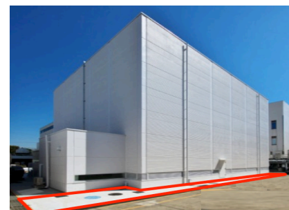
Fig-2 Application of Environmental-friendly Concrete to Earth Floor Concrete (denoted with red line)
