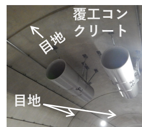
Photo-3: Joints of concrete lining
