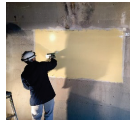
Testing of anti-spalling for tunnel lining concrete
