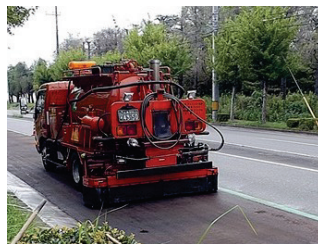
Pavement life extension with asphalt Emulsion
