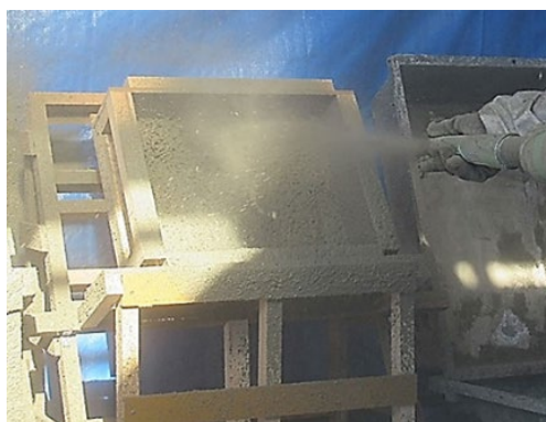
Photograph 1: Test of Spray injection patching
