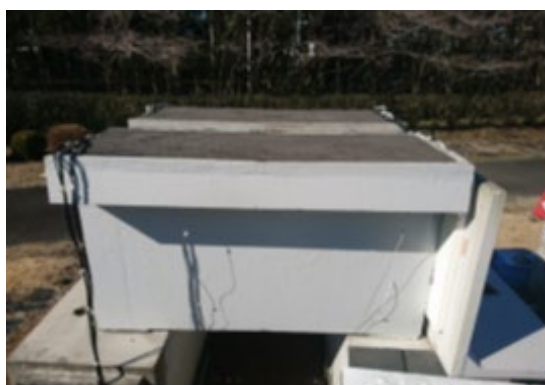
Photograph 3: Full-scale concrete girders with various surface protection materials
