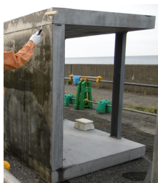
Photograph 1: Execution of surface-impregnation materials
