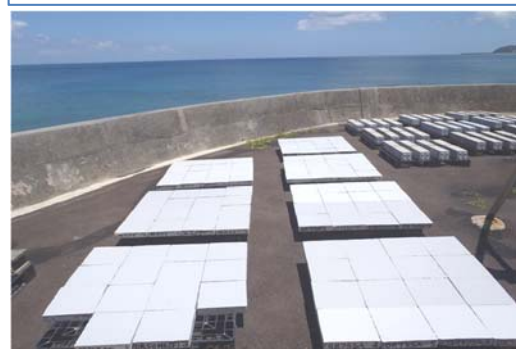
Exposure test of coating materials for concrete repair in Okinawa
